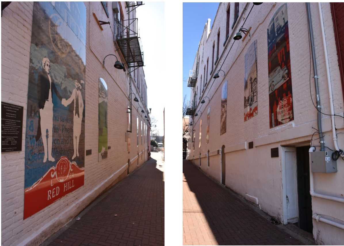
North elevation looking west (left) and east (right)
