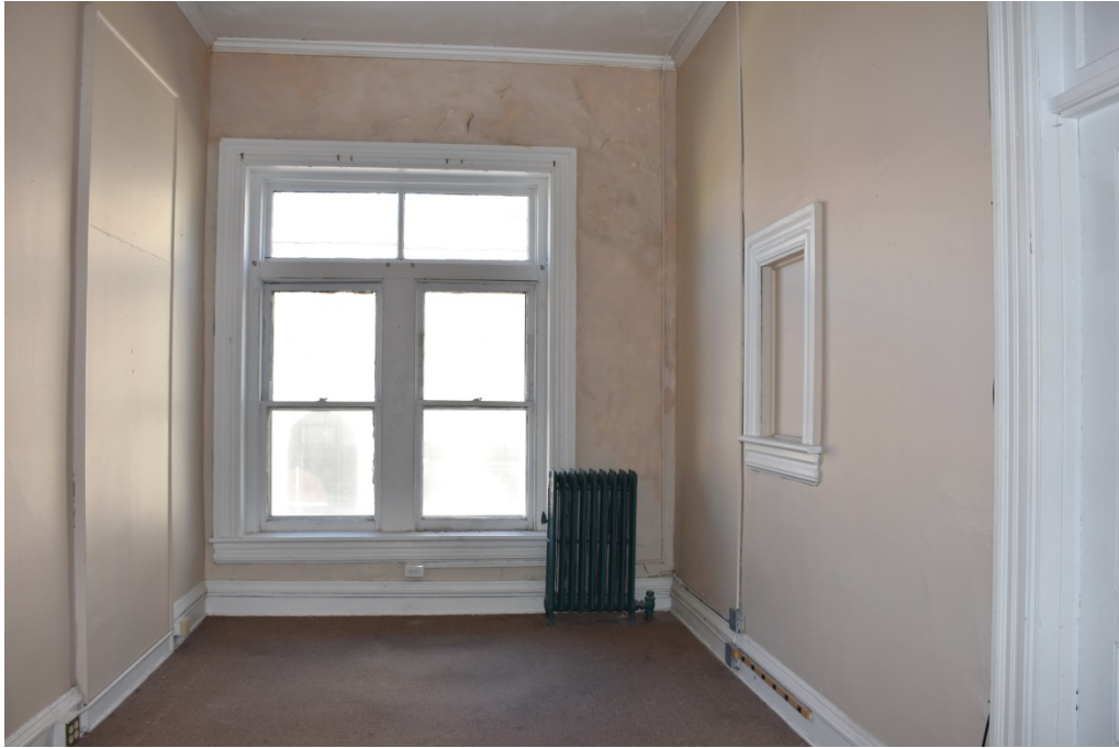
Northeast office 12, looking east (above)
